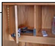
Upper security box with piano hinge
